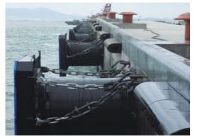
This chain is a versatile long link chain with a very high breaking strength. The chain is commonly used to secure fenders to docks but is popular also in many mooring and marine uses. The large internal dimensions of the links allow for the easy fitting of shackles and end fittings without the need of special end links.
