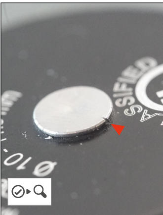
• Rivet slightly cracked
